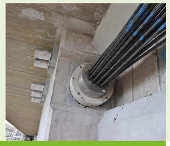
New steel cables fitted to the exterior of Clifton Bridge
