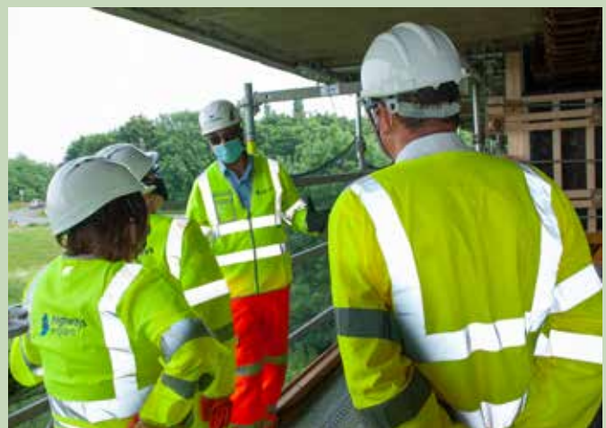
Explaining the Clifton Bridge Repair Scheme to Local MPs
